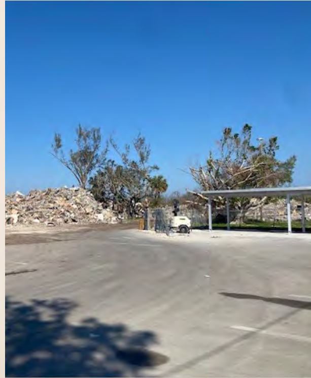
Historic Ft. Myers Beach Elementary School after Hurricane Ian, a current FEMA project.
