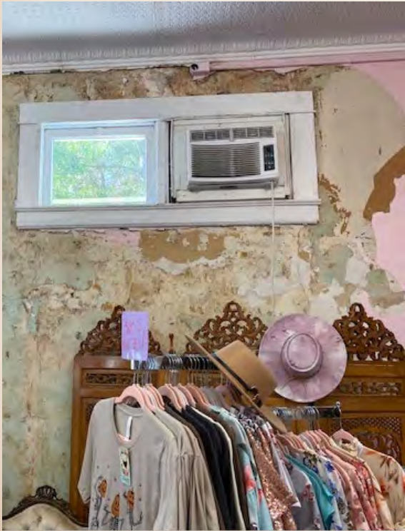
Sustained water damage at a store in Arcadia Main Street.
